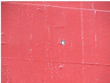
[93] [94] Reference point (metallic pin) on the wall, on the side of Rua Otávio Mendes
