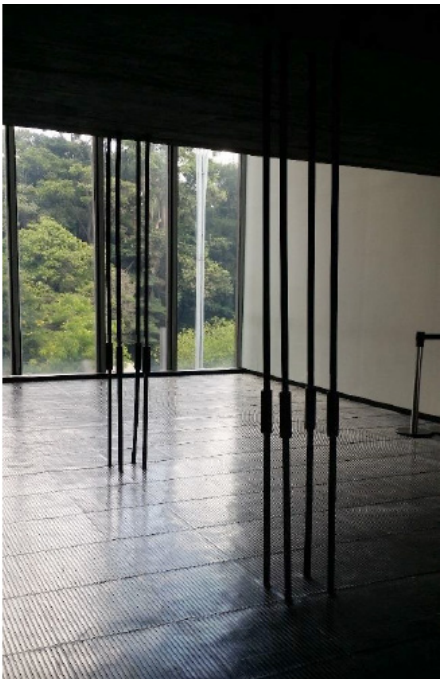
[98] [99] Misaligned or compressed tie rods
