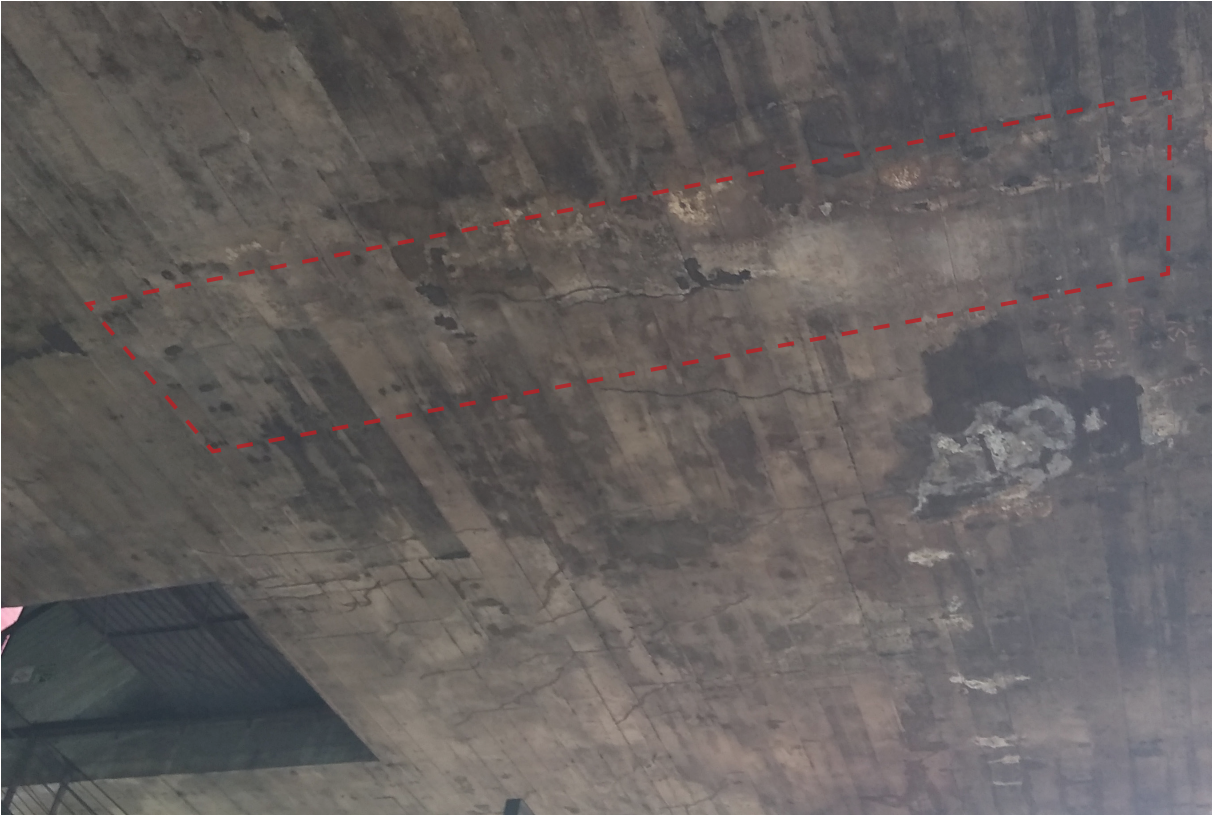
[82] Highlighted: cracks in beam V16
