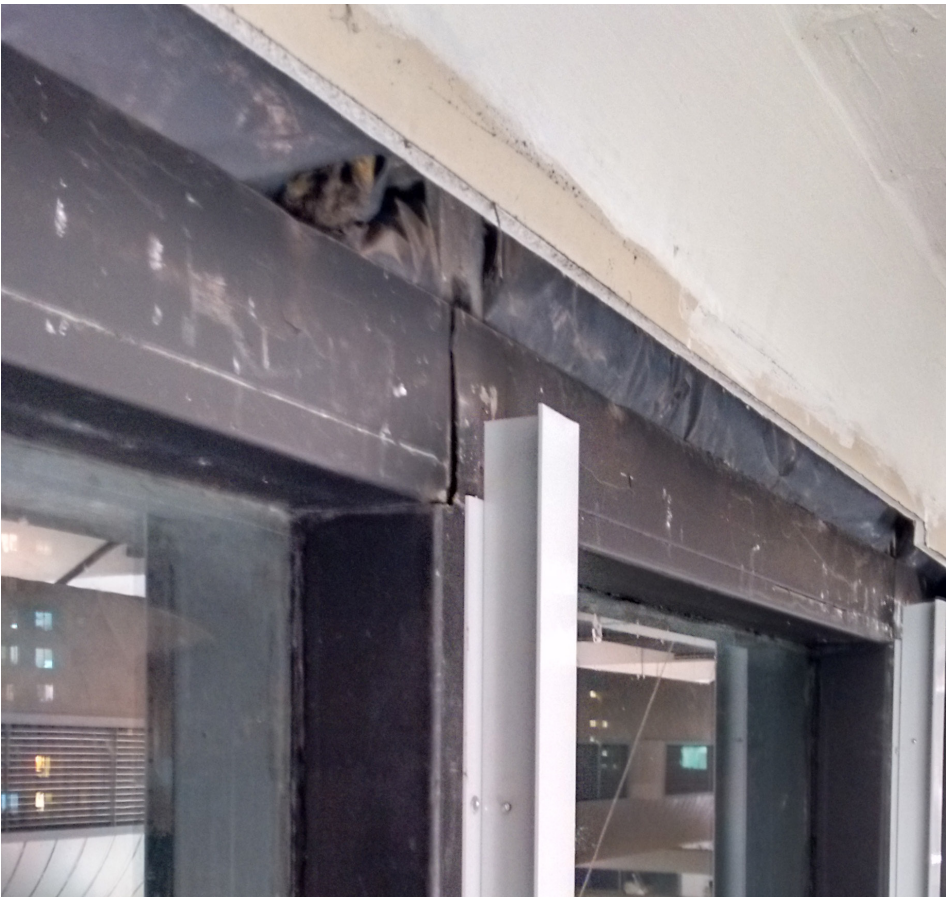
[100] Connection of the window casings with the roof slab
