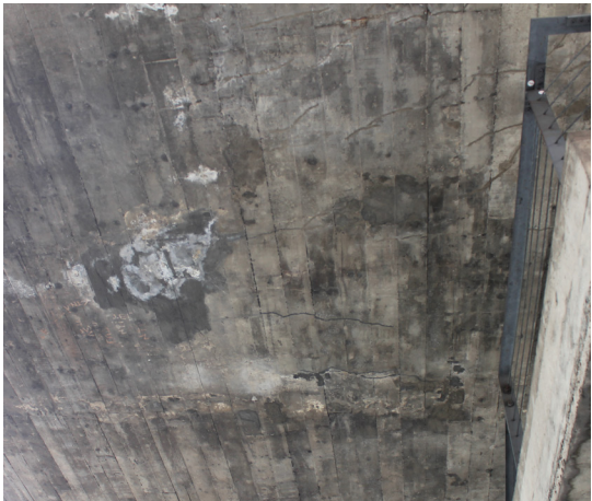
[83] [84] [85] Pathologies in the lower part of the first floor slab (ceiling of the plaza under the free span)
