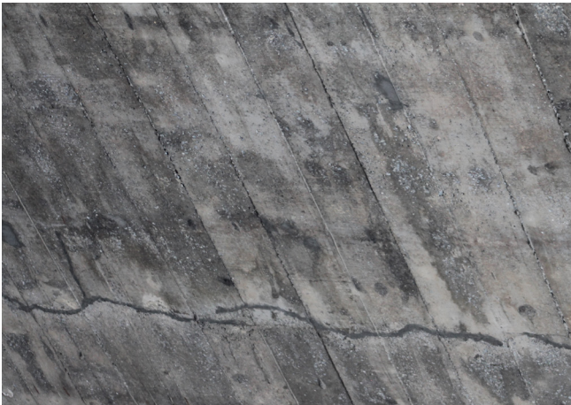
[83] [84] [85] Pathologies in the lower part of the first floor slab (ceiling of the plaza under the free span)
