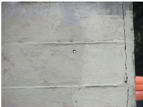
[93] [94] Reference point (metallic pin) on the wall, on the side of Rua Otávio Mendes
